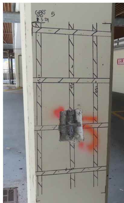
Photo 7. Column C-2 at Level Number 7
