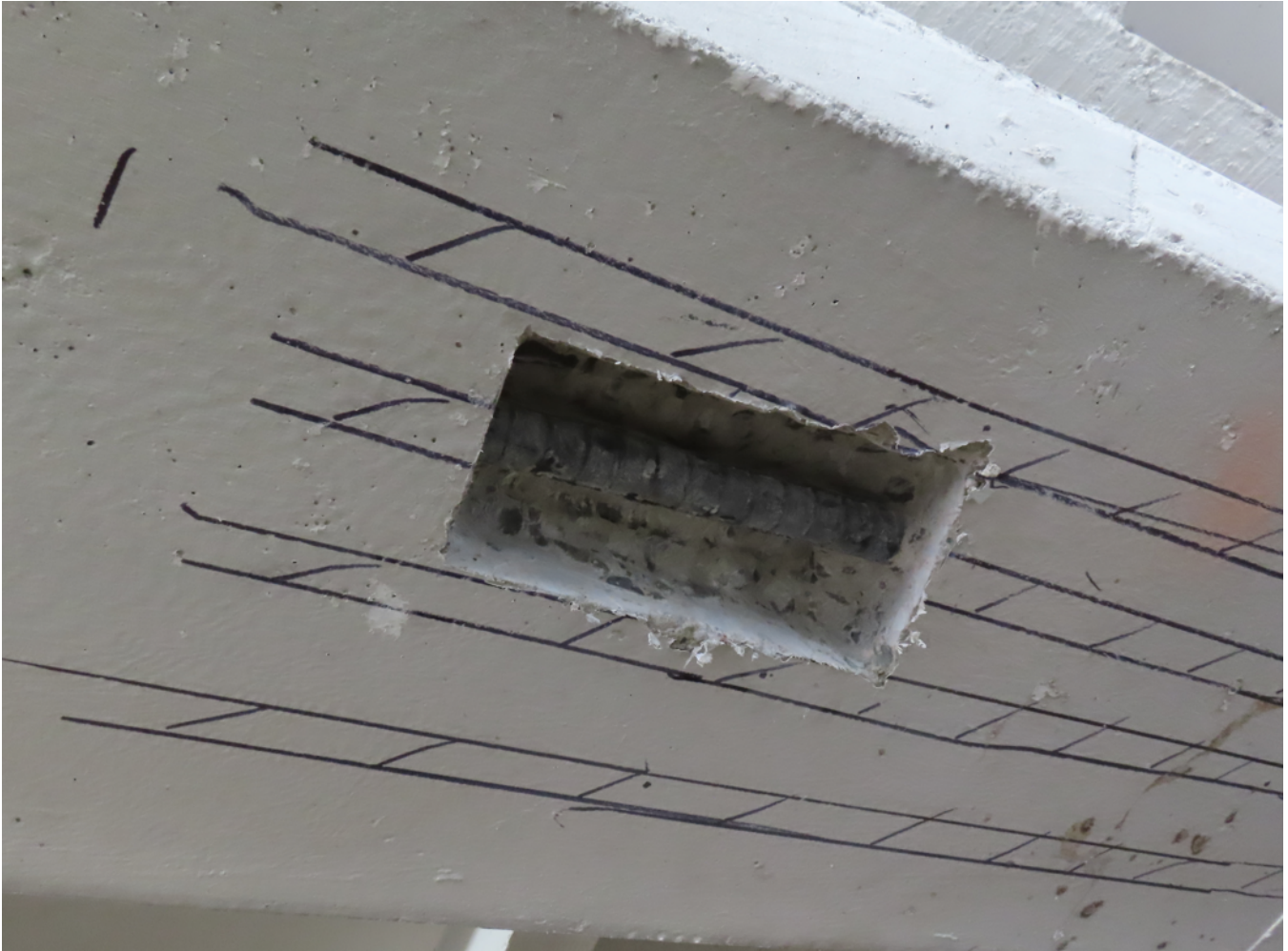
Photo 4. Bottom of Beam Grid 5, Between Grids C and D, Level Number 2
