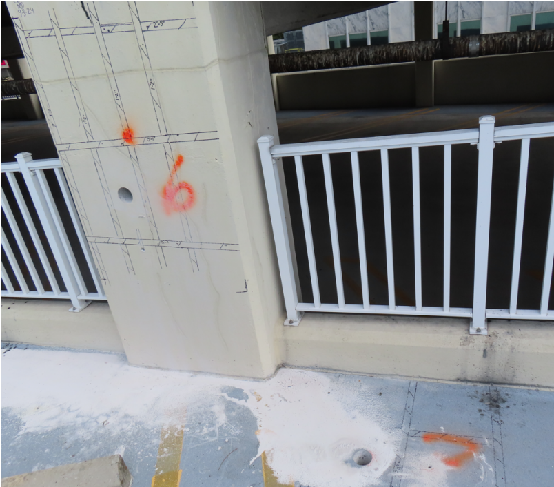
Photo 5. Column B-7 at Level Number 7
