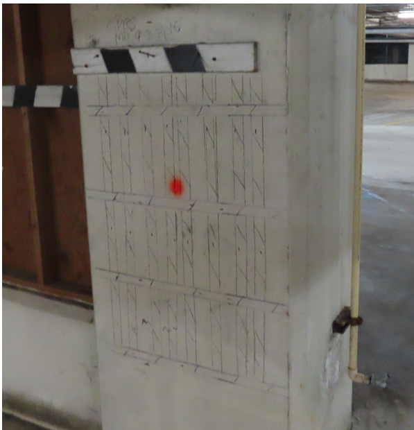
Photo 3. Column D-9 at Level Number 1
